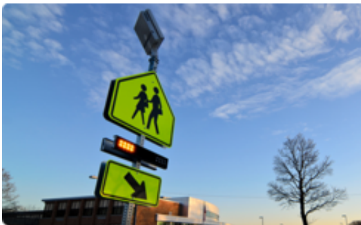
RRFB (Rectangular Rapid Flashing Beacon)
